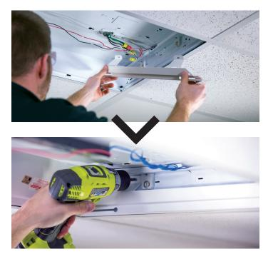
3. Optional: Install side plates (x2). This is dependent on whether or not there are gaps between the fixture and the existing ceiling grid.
