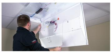
5. Hook safety cables into existing lances/holes of the fixture.
